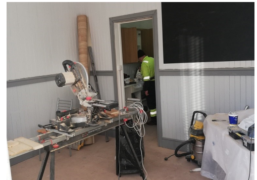
Getting There : New woodwork and paint
